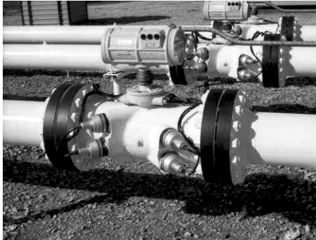
Figure 12-5 Transducers in this multipath ultrasonic meter are mounted so that the sound travel path crosses the pipe body at a set angle. Four pairs of transducers are used for high accuracy with many flow profiles.
